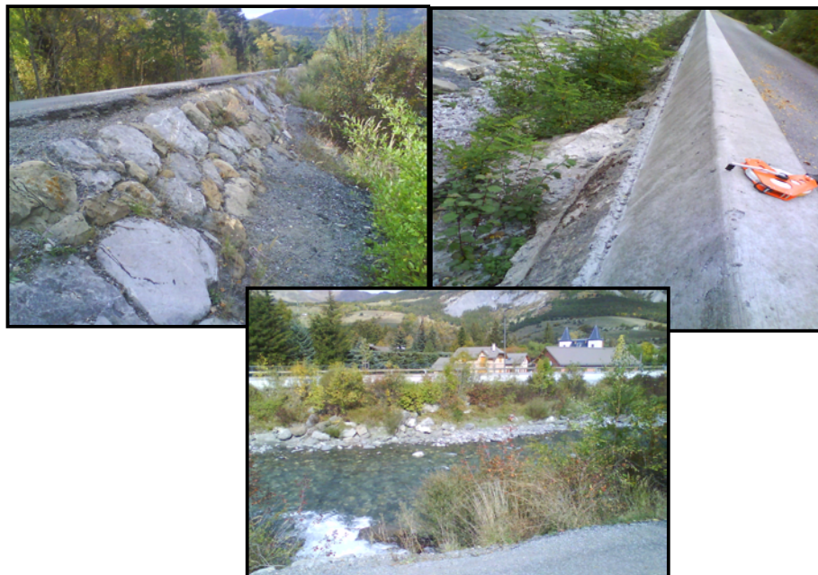
Figure 7: Flood embankments along Ubaye River
